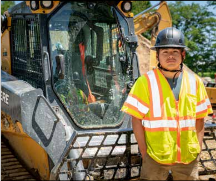
Kevin Coranado, Trainee, Operating Engineers Local 137 at the Westchester Joint Water Works site in Purchase, NY.
