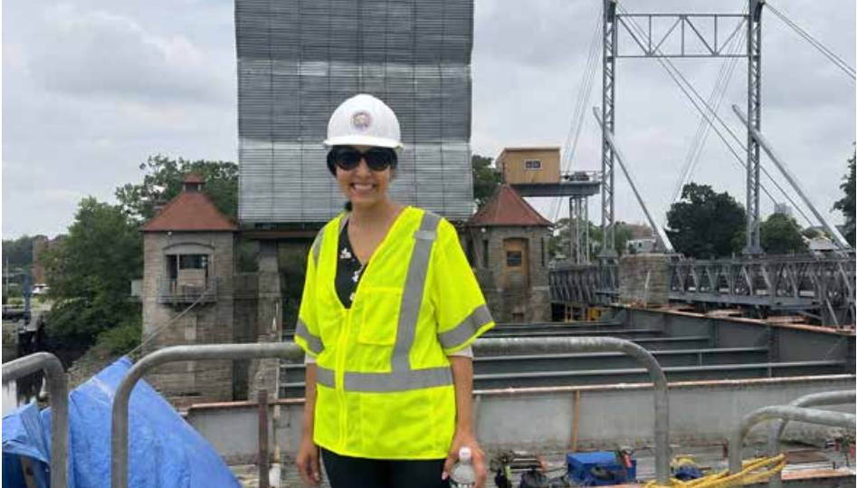
Susie Ghabour, P.E, at work on the Glen Island Bridge reconstruction project for the Westchester County Department of Public Works and Transportation
