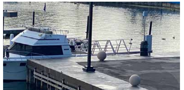
Increased awards will help marinas continue to install new pump out stations, modernize aging equipment, purchase pump out boats and maintain existing facilities.
