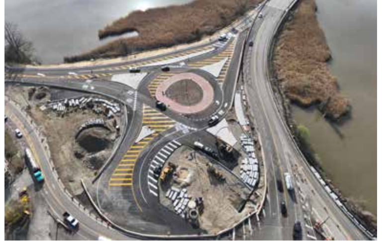
An aerial view of the Annsville Circle roundabout in Cortlandt Manor, NY.
