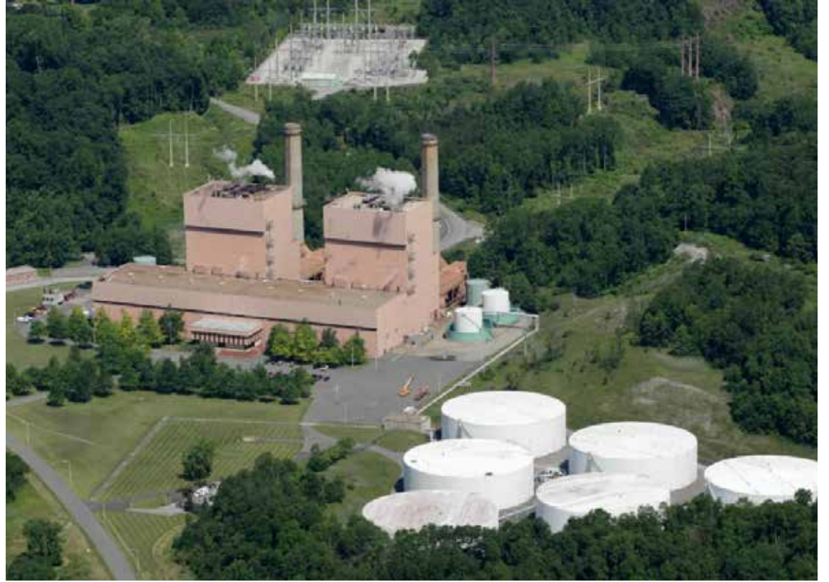
The Roseton energy plant in the Town of Newburgh.
