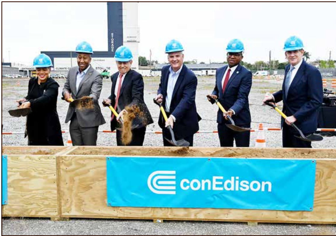
Con Edison's Chairman and Chief Executive, Tim Cawley (center), leads the groundbreaking for the Reliable Clean City – Idlewild Project in Jamaica, Queens. Joining him, from left were: Con Edison Vice President LaAsia Hundley, New York State Assembly Member Clyde Vanel, Port Authority Executive Director Rick Cotton, Queens Borough President Donovan Richards Jr., and MTA Chair and CEO Janno Lieber.
