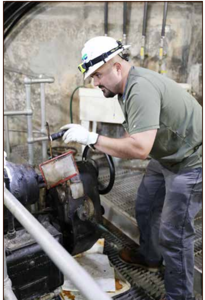
DEP's Ross Fratto closes the first of six water lines.
