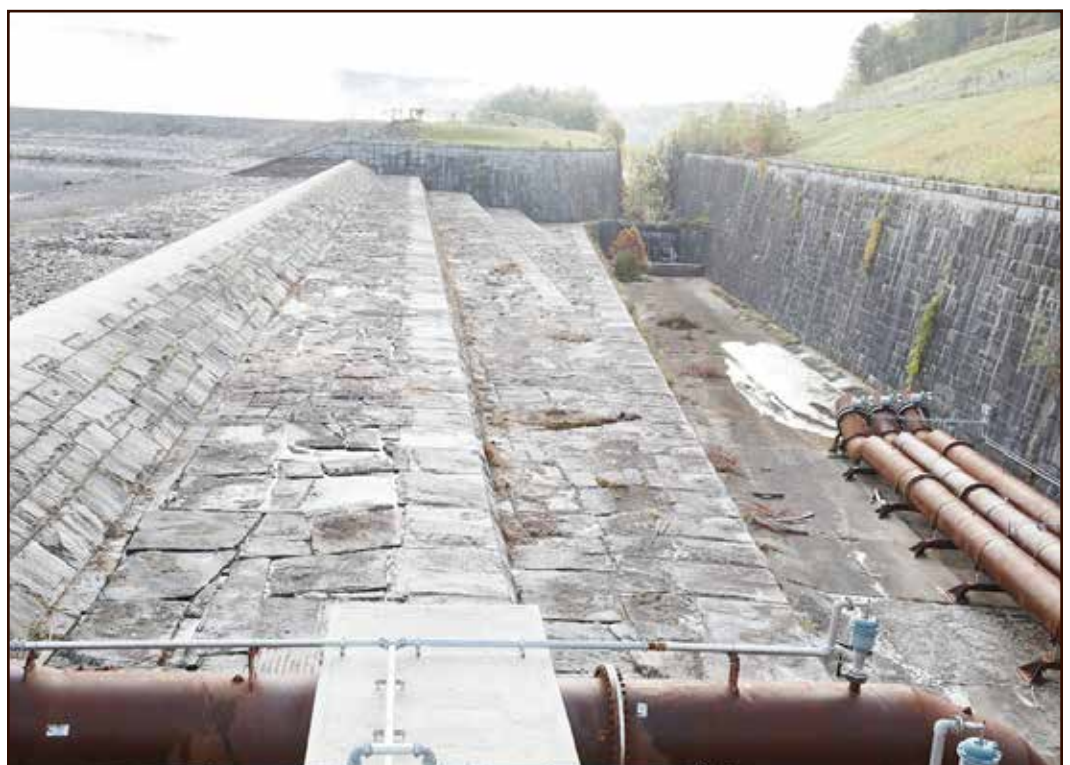
Siphons at the Rondout Reservoir were installed to enable the release of water from the reservoir into the Rondout Creek during the Delaware Aqueduct Repair Project.
