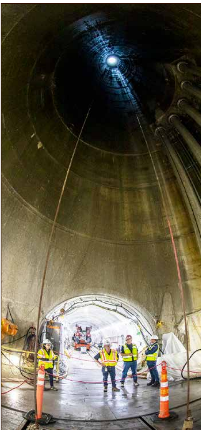
DEP Commissioner Rit Aggarwala visits the shaft in Wappinger on Sept.13. From right, DEP Commissioner Rit Aggarwala, Executive Director in the Bureau of Engineering Design and Construction Sean McAndrew, Director of External Affairs John Milgrim, and Deputy Commissioner of the Bureau of Public Affairs and Communications Beth DeFalco.
