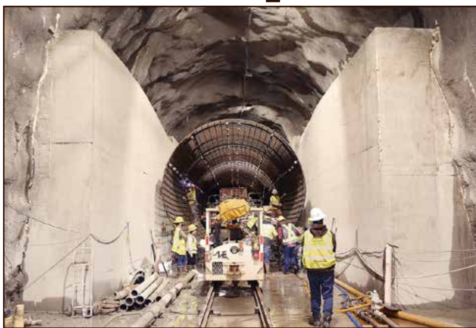
Work has begun on the final phase of the Delaware Aqueduct repair project. The bypass tunnel is lined with multiple layers of steel, rebar and concrete, making it extremely robust. Photo Credit/NYCDEP
