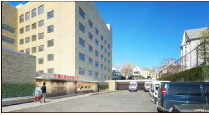
Part of the plan includes an expansion of the Emergency Department at Montefiore Mount Vernon Hospital.
