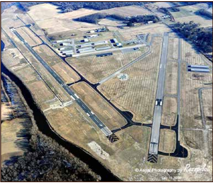
An aerial view of Orange County Airport in Montgomery, NY.
