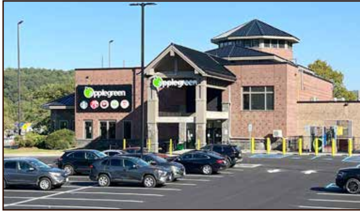
The renovated Sloatsburg Service Area on the New York State Thruway reopened with a host of new retail tenants.
