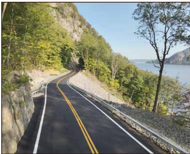
ECCO III Enterprises of Yonkers, NY was the contractor that worked on the Storm King Highway project in Orange County.
