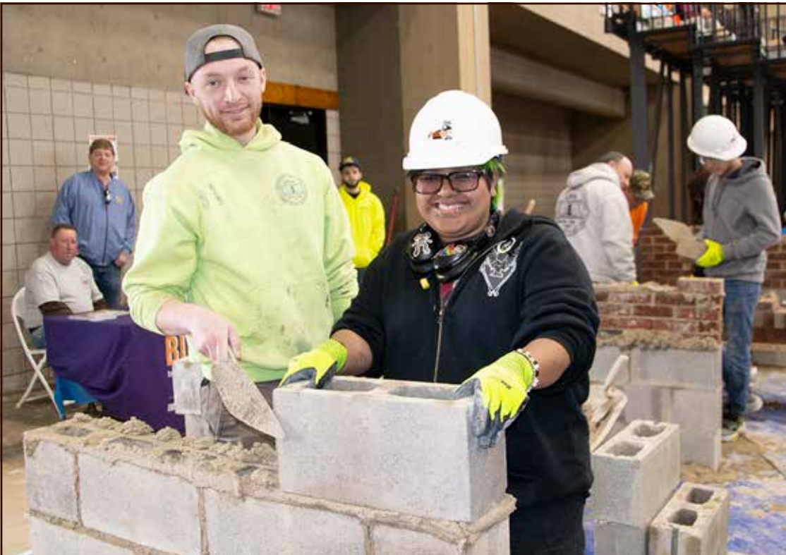
Raven Astudillo, a junior at Roosevelt High School in Yonkers, received pointers in laying concrete block from instructor Chris Brozowski of Bricklayers Local 1 at the Hudson Valley Construction Career Day in Rockland County in March 2023.
