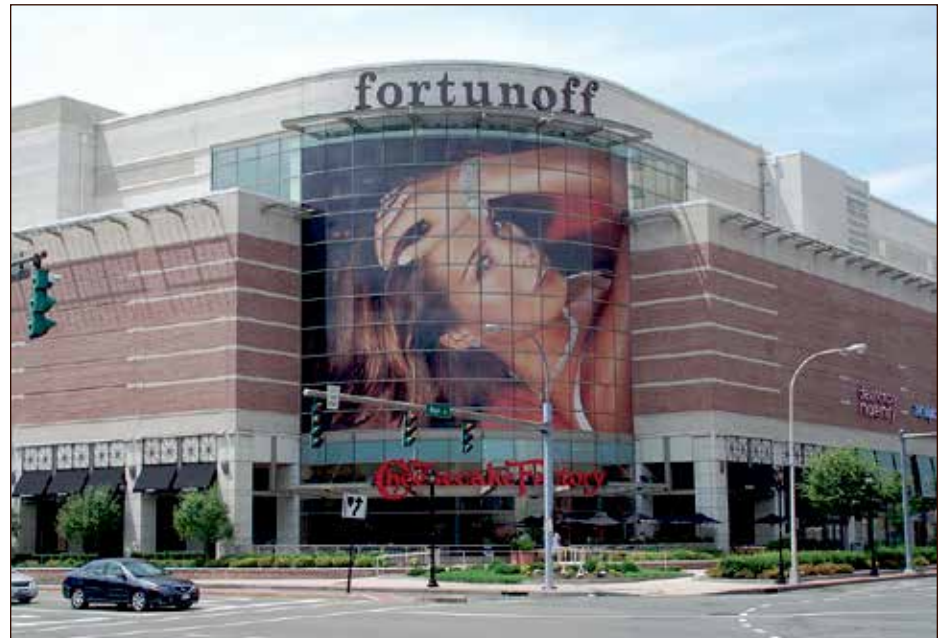
Fortunoff Building where Darante Construction served The Whiting-Turner Contracting Company providing masonry work.
