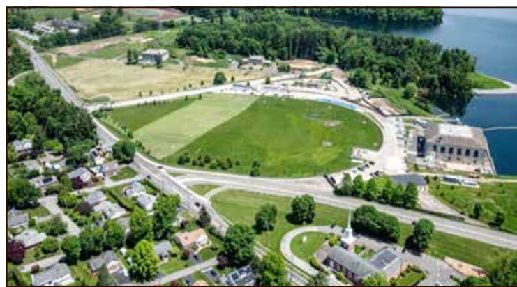
The Kensico Campus in Valhalla, NY, will be the site of a new electrical building, major modifications and construction of connecting shafts and connecting tunnel for the drinking water from the Kensico Reservoir.
