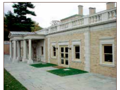
Sleepy Hollow Country Club in Scarborough, NY where Darante Construction completed masonry work.
