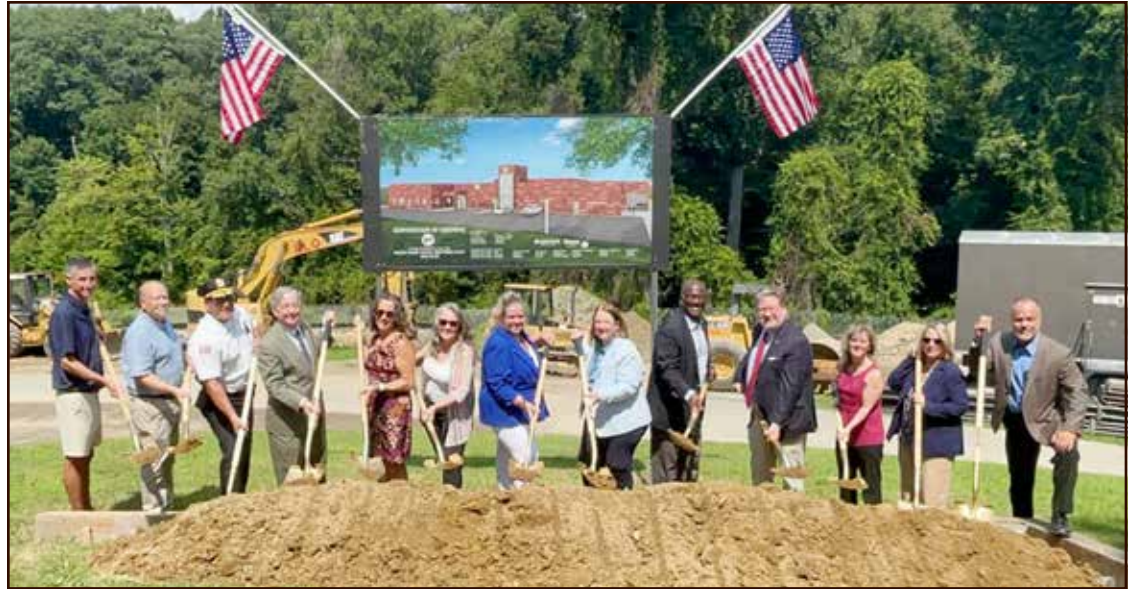
Village and Town of Ossining officials were joined recently by county and state government representatives to celebrate the official groundbreaking for the new Indian Brook Water Treatment Plant. The $100-million project is the largest infrastructure project in Ossining's history and one of the largest municipal capital projects in memory in the region.
