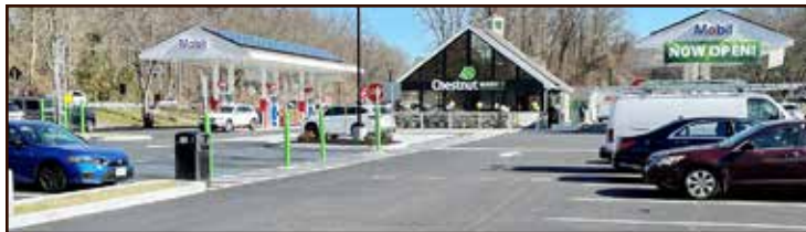
The fully renovated service area located between Exit 13 (Mamaroneck Avenue) and Exit 14 (North Street) in the City of White Plains on the Hutchinson River Parkway.
