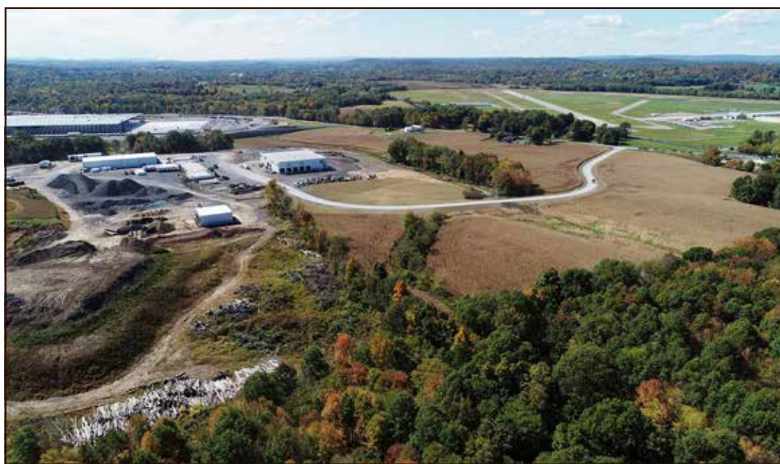
An aerial of the Aden Brook Business Park site in Montgomery, NY.
