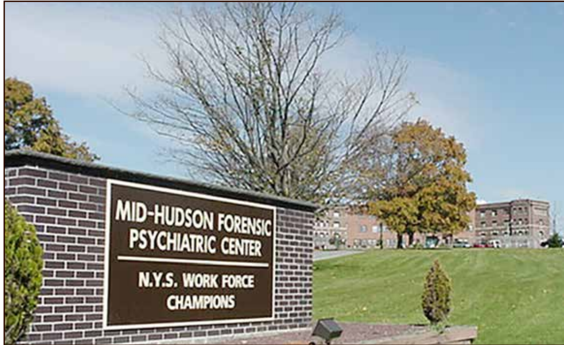
Work is expected to begin soon on a major redevelopment of the Mid-Hudson Psychiatric Center in New Hampton in Orange County.
