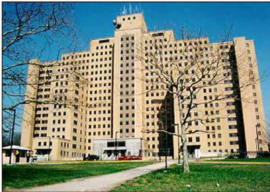
The Creedmoor Community Master Plan introduces approximately 2,800 units of new housing, with more than 55% designated as homeownership.
