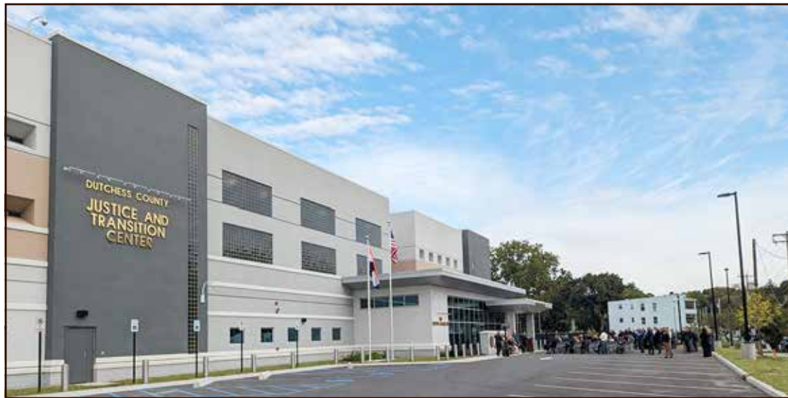
The construction of the new Dutchess County Justice & Transition Center was performed under a Project Labor Agreement.
