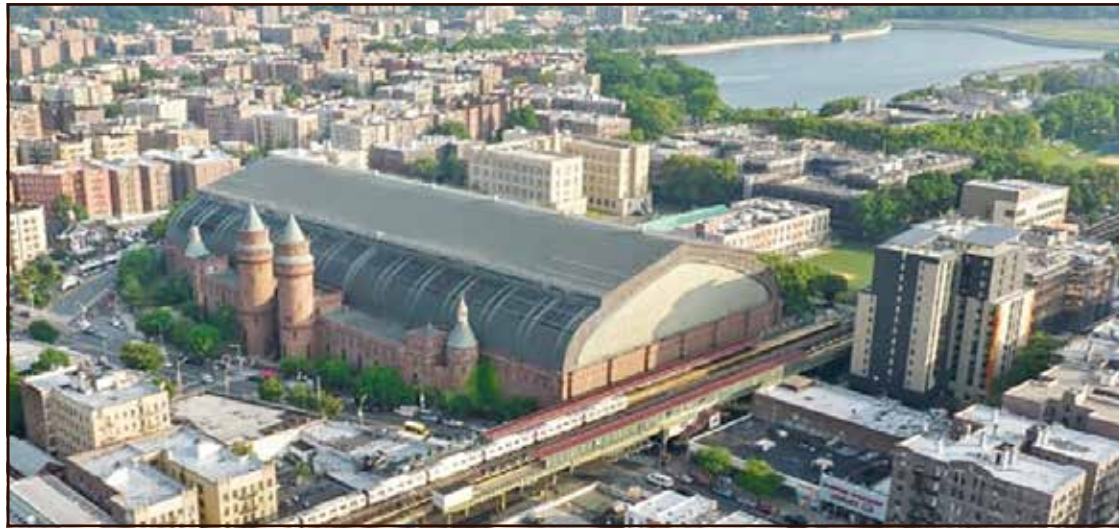
One of the few remaining armories in New York City, the Kingsbridge Armory, opened in 1917 and was used throughout the first half of the 20 th century. Designated as a New York City Landmark in 1974, the Armory was listed on the New York State and the National Register of Historical Places in 1982. The Armory was transferred to the City of New York in 1996.
