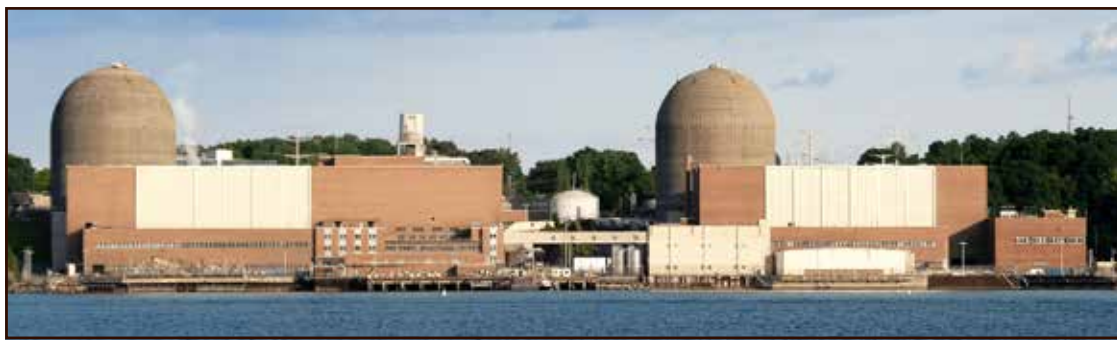
All 3,998 spent fuel assemblies are now contained within 127 reinforced concrete and steel casks on the Indian Point site's independent spent fuel storage installations.
