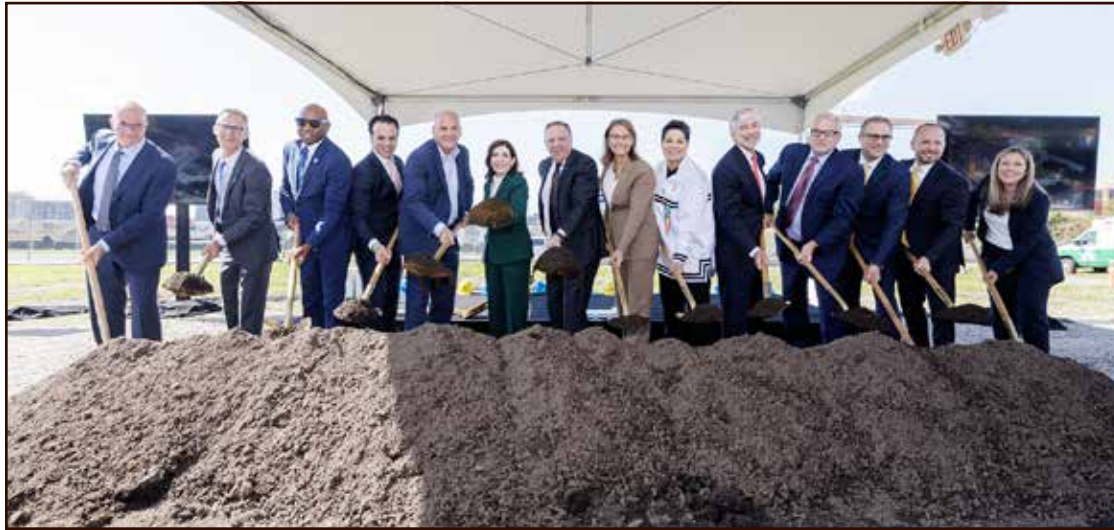
Gov. Kathy Hochul was joined by federal officials, the Premier of Quebec and representatives of Transmission Developers and Hydro-Quebec at the Sept. 19 groundbreaking of a converter station in Astoria, Queens for the 339-Mile Champlain Hudson Power Express transmission line.
