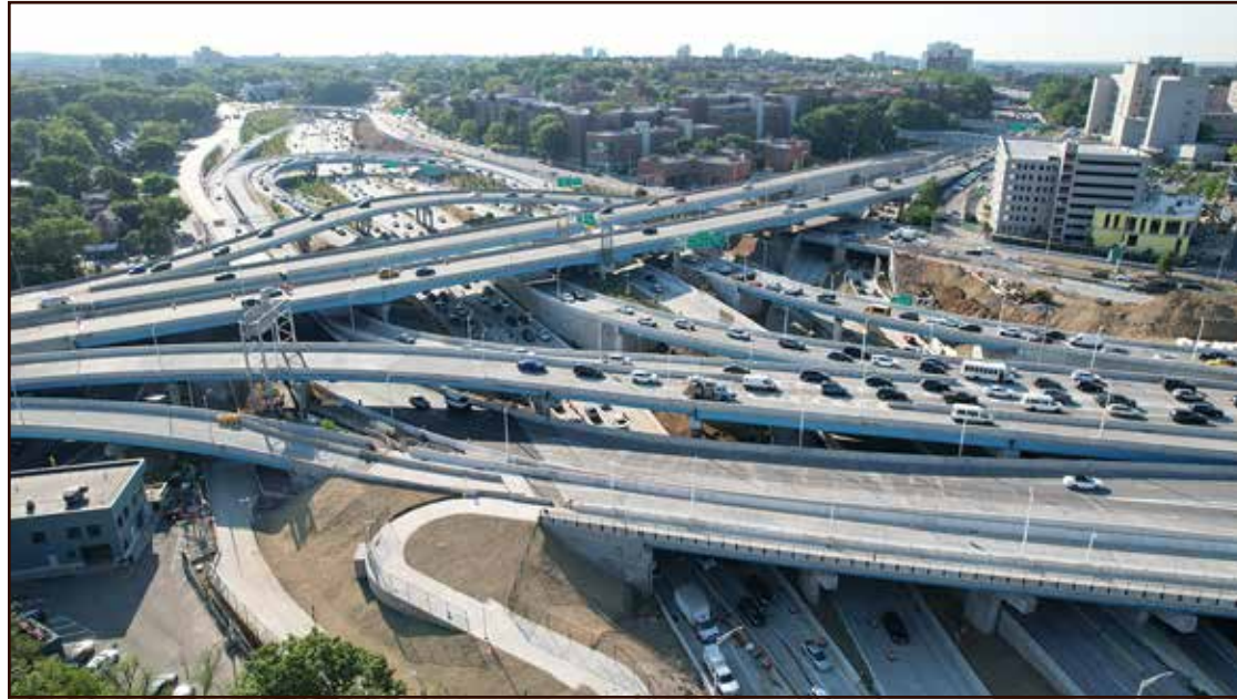
The completed Kew Gardens Interchange in Queens, NY.
