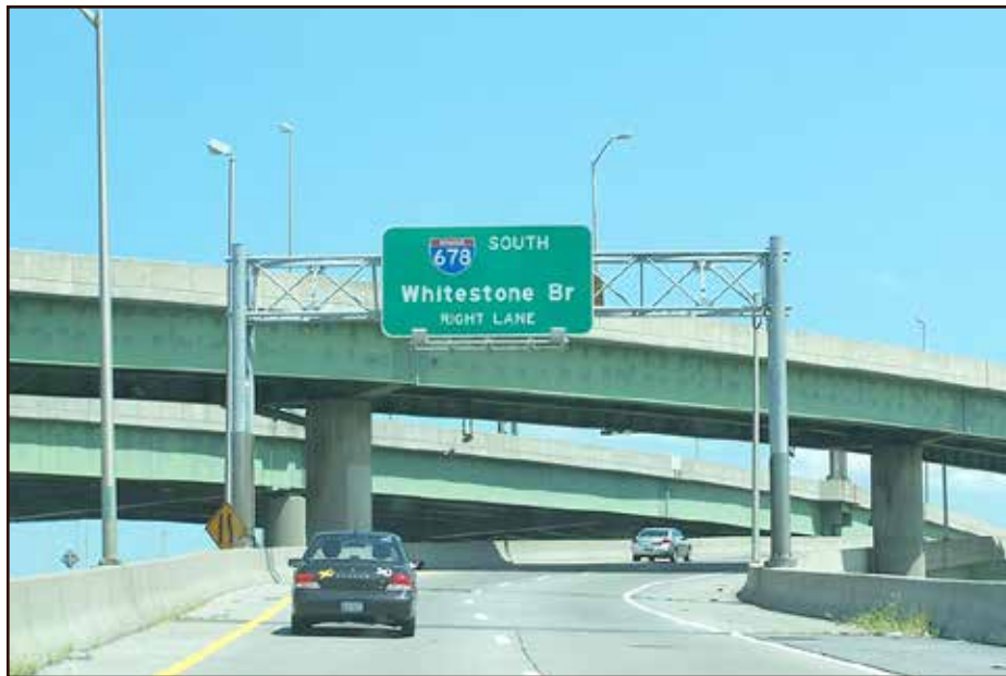
Construction has begun on the nearly $45-million Bruckner Expressway bridge project.
