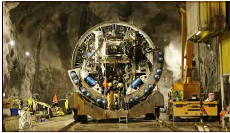
Tunnel Boring Machine used for work on the Delaware Aqueduct.
