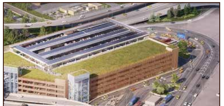
The design-build project at JFK International Airport consists of the design and construction of the on-airport roadway transportation network.
