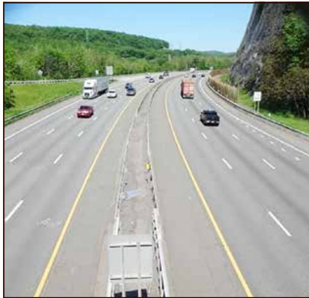
A section of the New York State Thruway near the Rockland and Orange County line.
