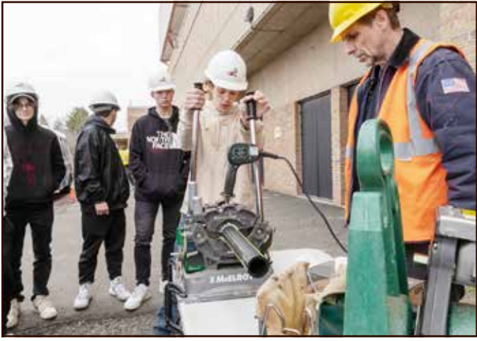
Students take turns at compaction.
