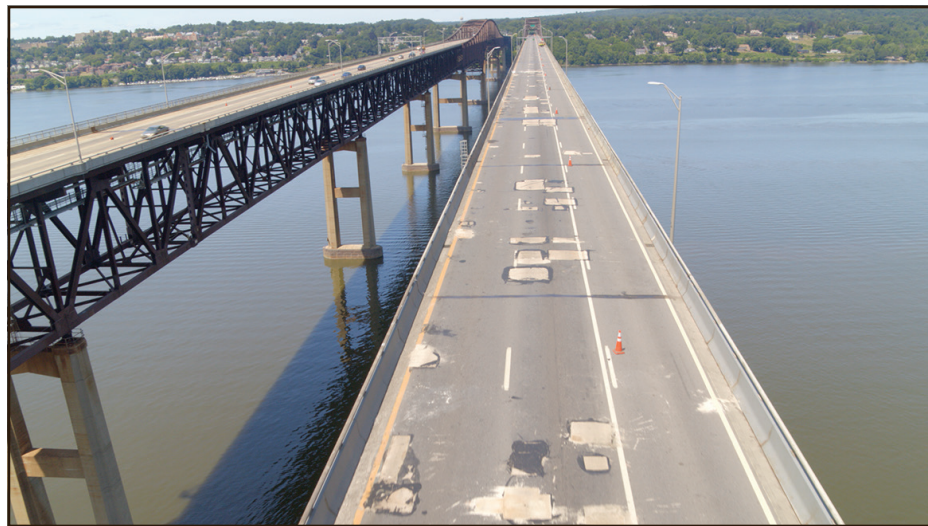
A look at current deck conditions on the Newburgh-Beacon Bridge's north span. The span will experience a complete deck replacement, set to be complete by 2023.
